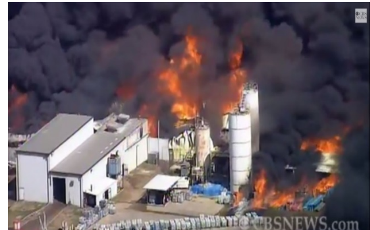
Magnablend Fire, Texas, 2011
